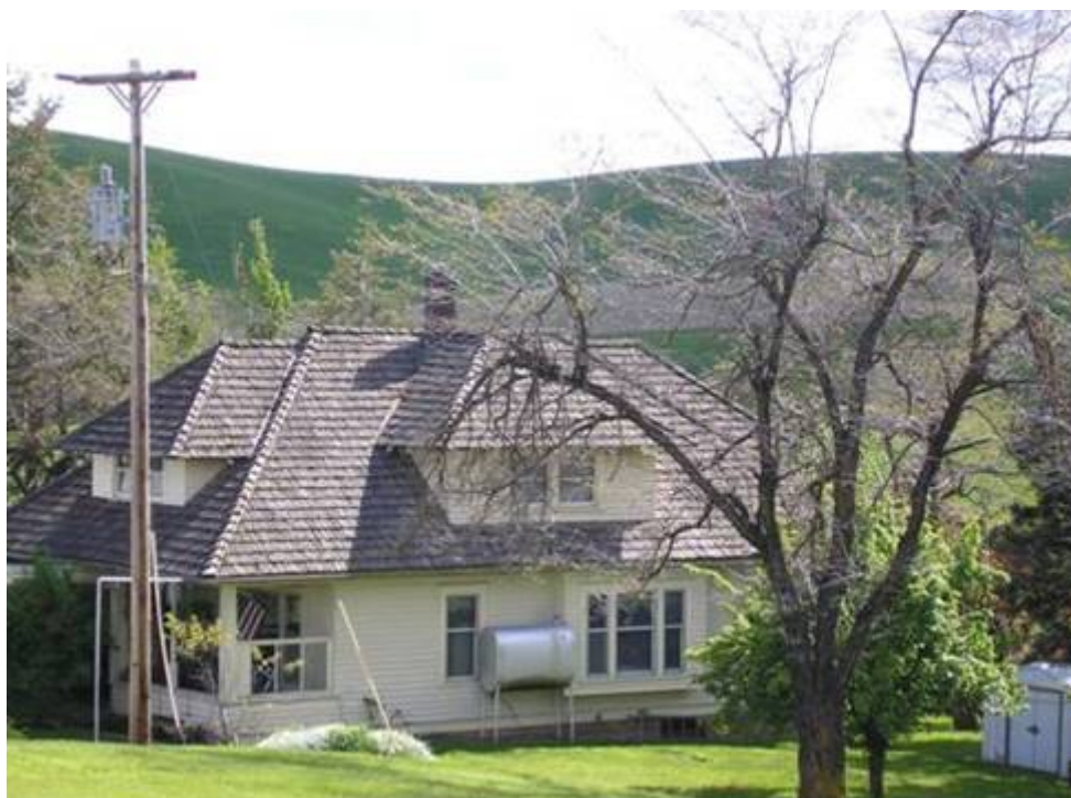
Heating oil tank (AST)
