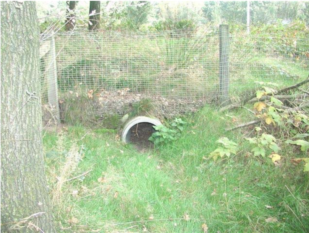
Figure 2. Badger tunnel with small animal fencing (Netherlands). Suitable for small mammals, reptiles or amphibians. Author recommends 36" or 48" box culverts for common mid-sized species.
